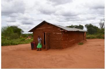
The church here is a small mud building about 15x30. The walls are red mud packed into a lattice of sticks with the ever-present corrugated iron roof. Dirt floor, no windows, and a makeshift door – this is not your standard, everyday church like we would expect in America. This is the evidence of desperate faith and a desire to worship God where it is not convenient.
